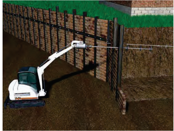
Figure 1.42 Rendering of helical tieback installation for soldier pile and timber lagging wall
