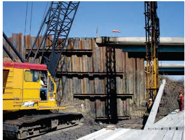
Figure 1.43 Multi-tier helical tieback installation to support sheet pile wall
