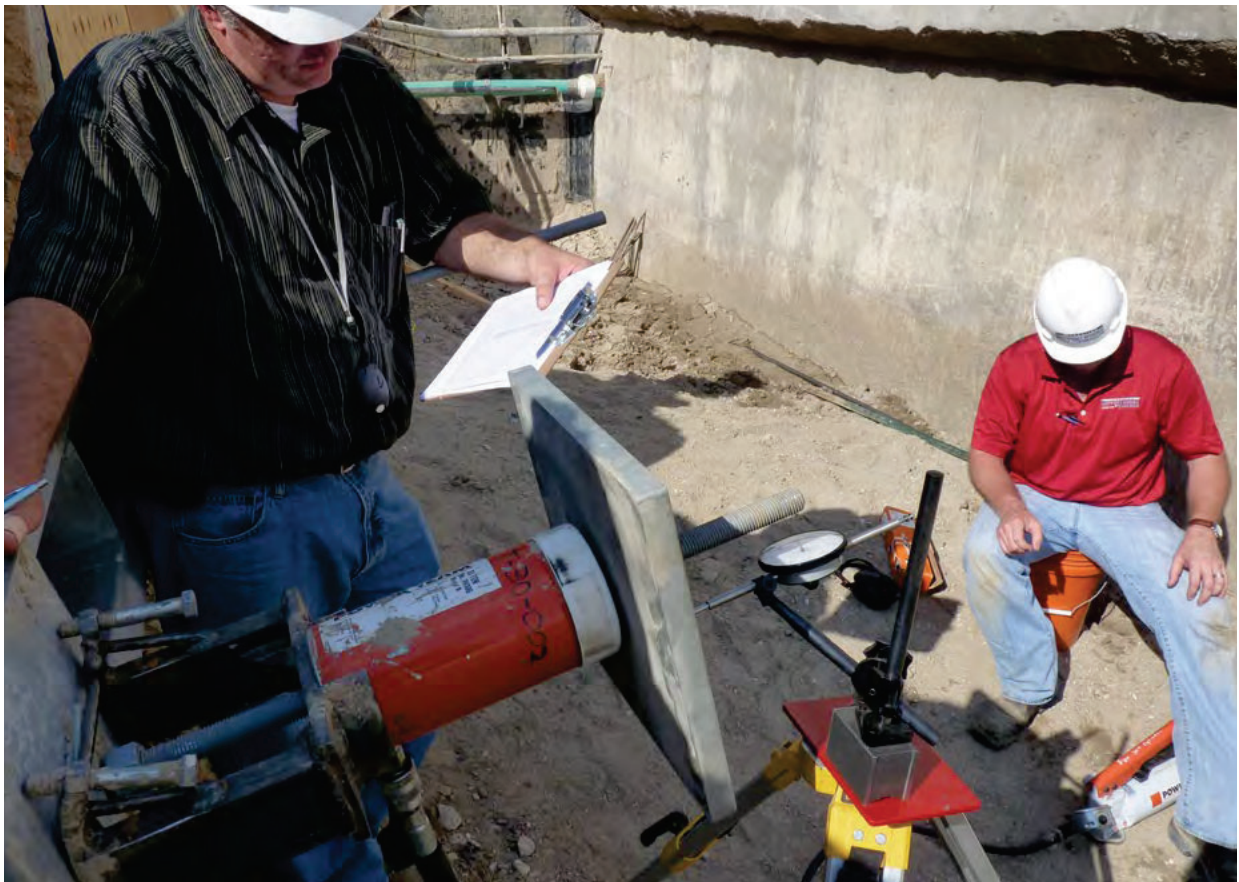
Figure 1.49 Pretensioning helical tieback
