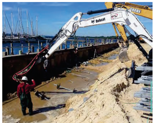
Figure 1.44 Helical tiebacks stabilize marina seawall
